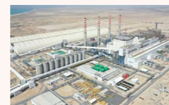
Hassyan Power Plant in Dubai
